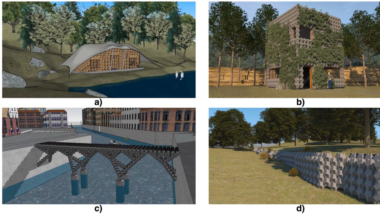
**Fig. 2.** Prototypical droxel structures: (a) timber droxel shelter, (b) concrete droxels multi-story house, (c) concrete droxel footbridge, (d) plastic or concrete droxel retaining wall.
