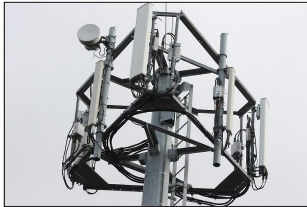
**Figure 1.5:** Configuration of sector antennas for cellular communication [2].
